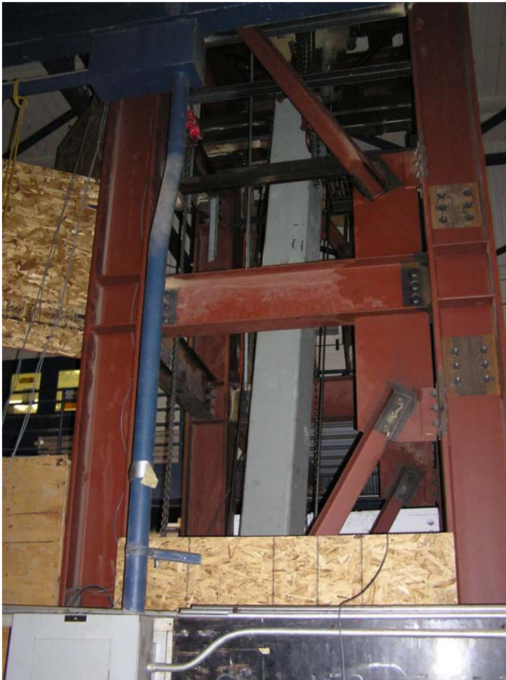
Figure 1 – Buckling Restrained Brace attached to the loading frame
